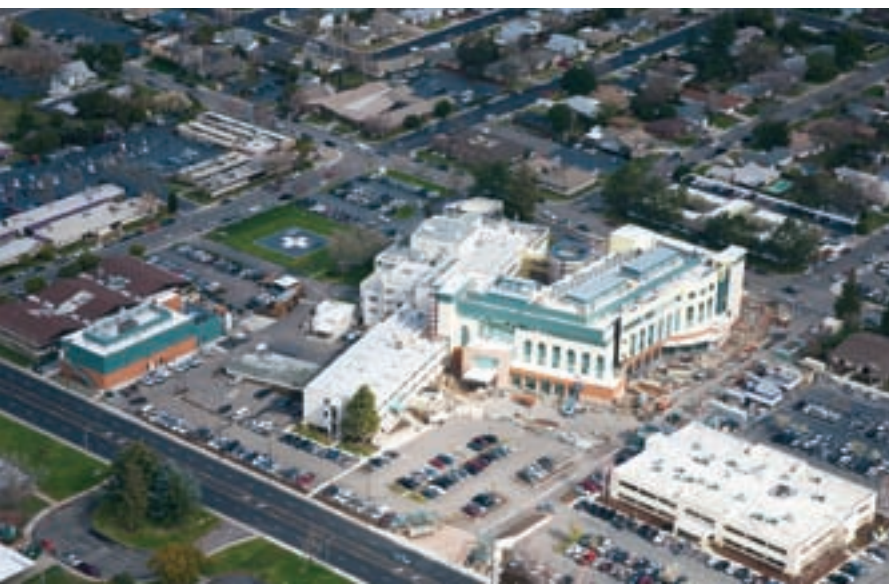
The new central utility plant, is now ready to supply power to the entire facility.
