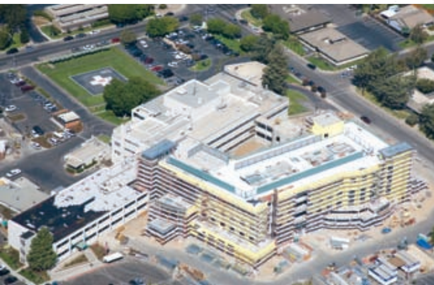
The four-story, 90-bed South Wing should finish construction by Fall, 2009.
