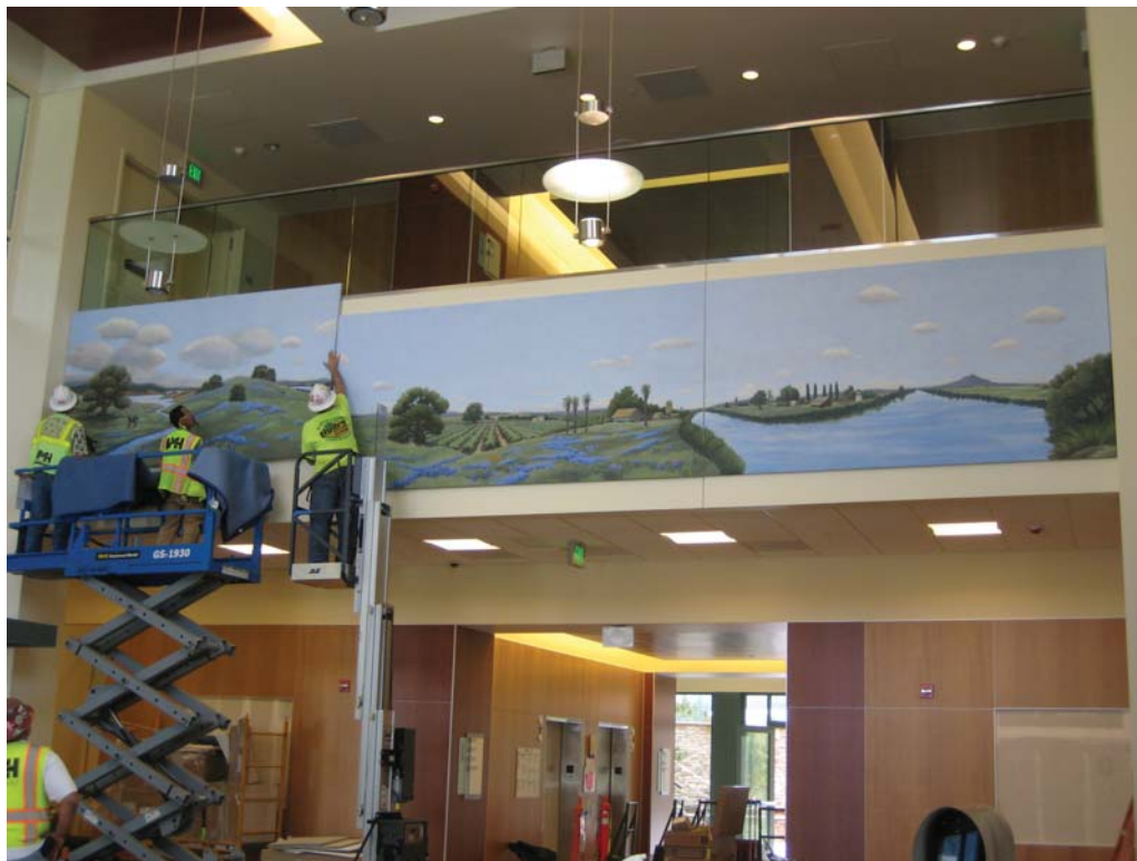
South Wing main lobby mural installation. The mural weighed about 200 pounds.
